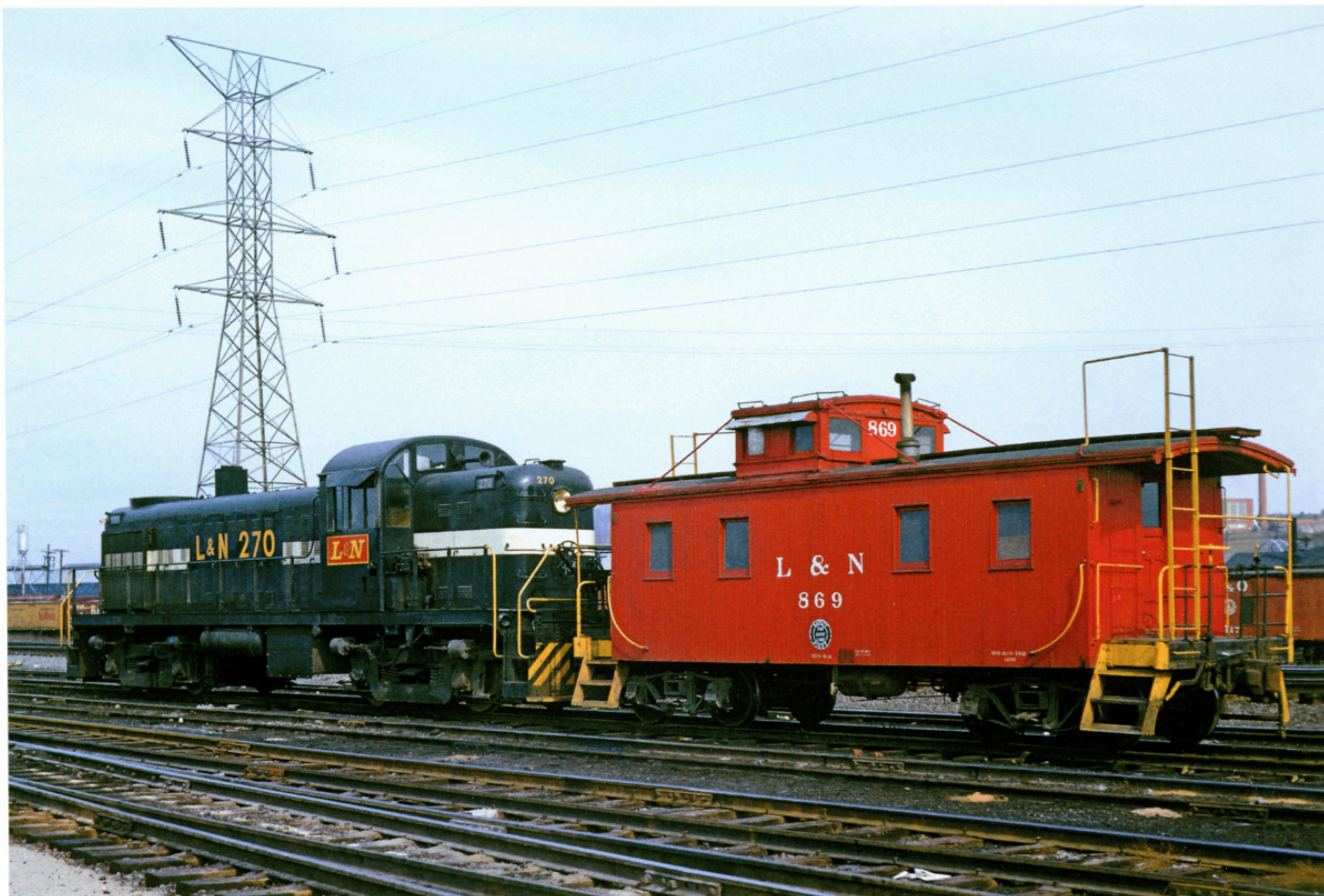
Pictured at the B&O Storrs yard in Cincinnati in 1963, former Lehigh & New England RS-2 270 (ex-L&NE 661) has just completed a transfer run from DeCoursey. Ancient wooden cupola caboose 869 was still equipped with arch-bar trucks, plus four stabilizing braces on all four corners of the cupola. Heavy slack action could deflect a cupola considerably — not to mention what it would do to its occupants! — F. M. Bowden photo
