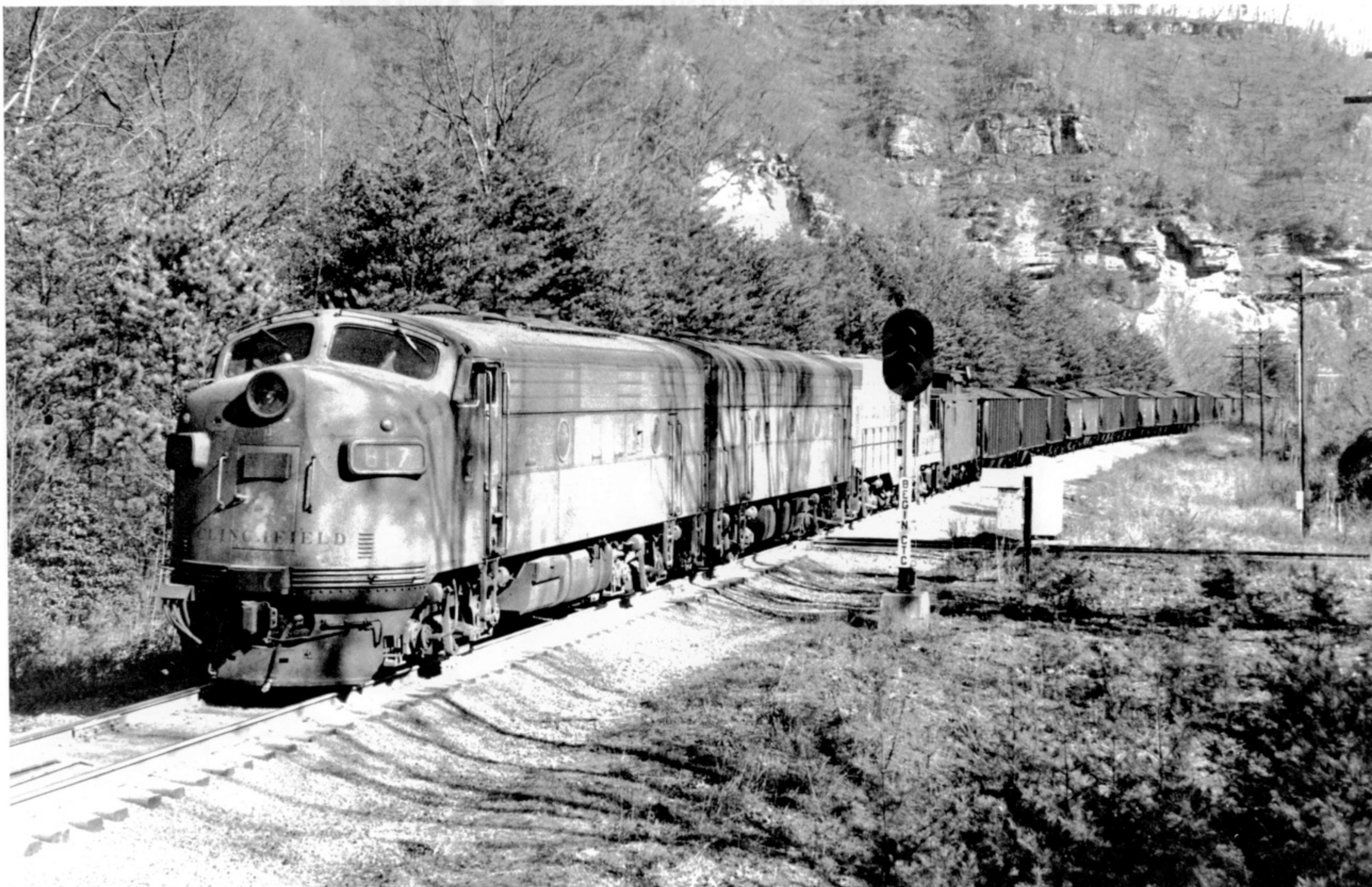
Clinchfield 817 plus two assistants add their tractive effort on the rear of a southbound coal train at Pool Point, just south of Elkhorn City, Kentucky on December 15, 1964. The head end of the train is already in Virginia. The pusher units will stay on until the grade eases at Towers. (Ron Flanary Photo)
