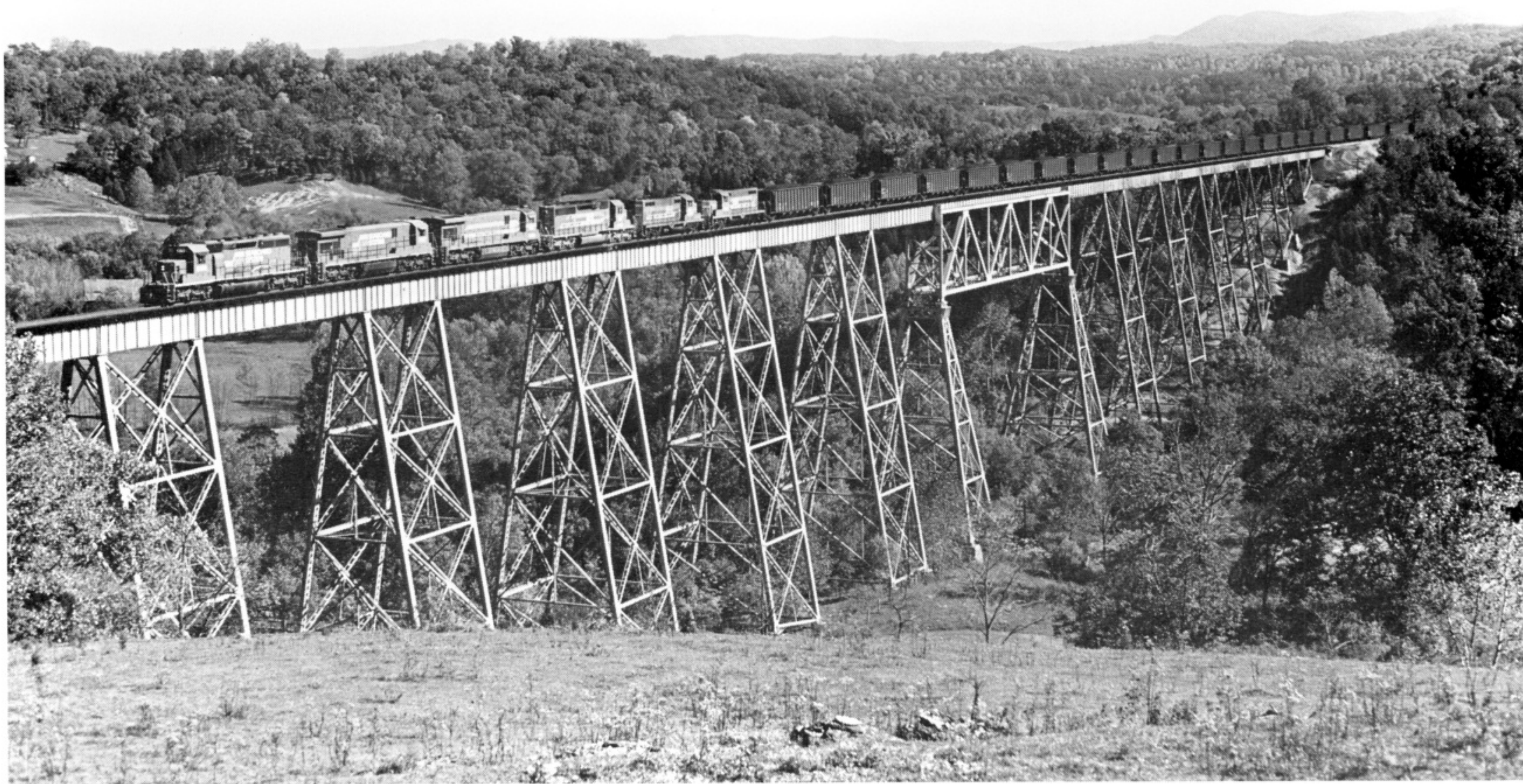
A northbound coal train rides high across Red River Viaduct at Sloan, Kentucky on the former Eastern Kentucky Division. The 233 foot high structure helped maintain a steady .4 percent grade on the Ravenna to Patio line. This October 19, 1986 unit coal train appears amply powered, with a generous mixture of EMD and GE four and six-axles. (Jill Oroszi)
