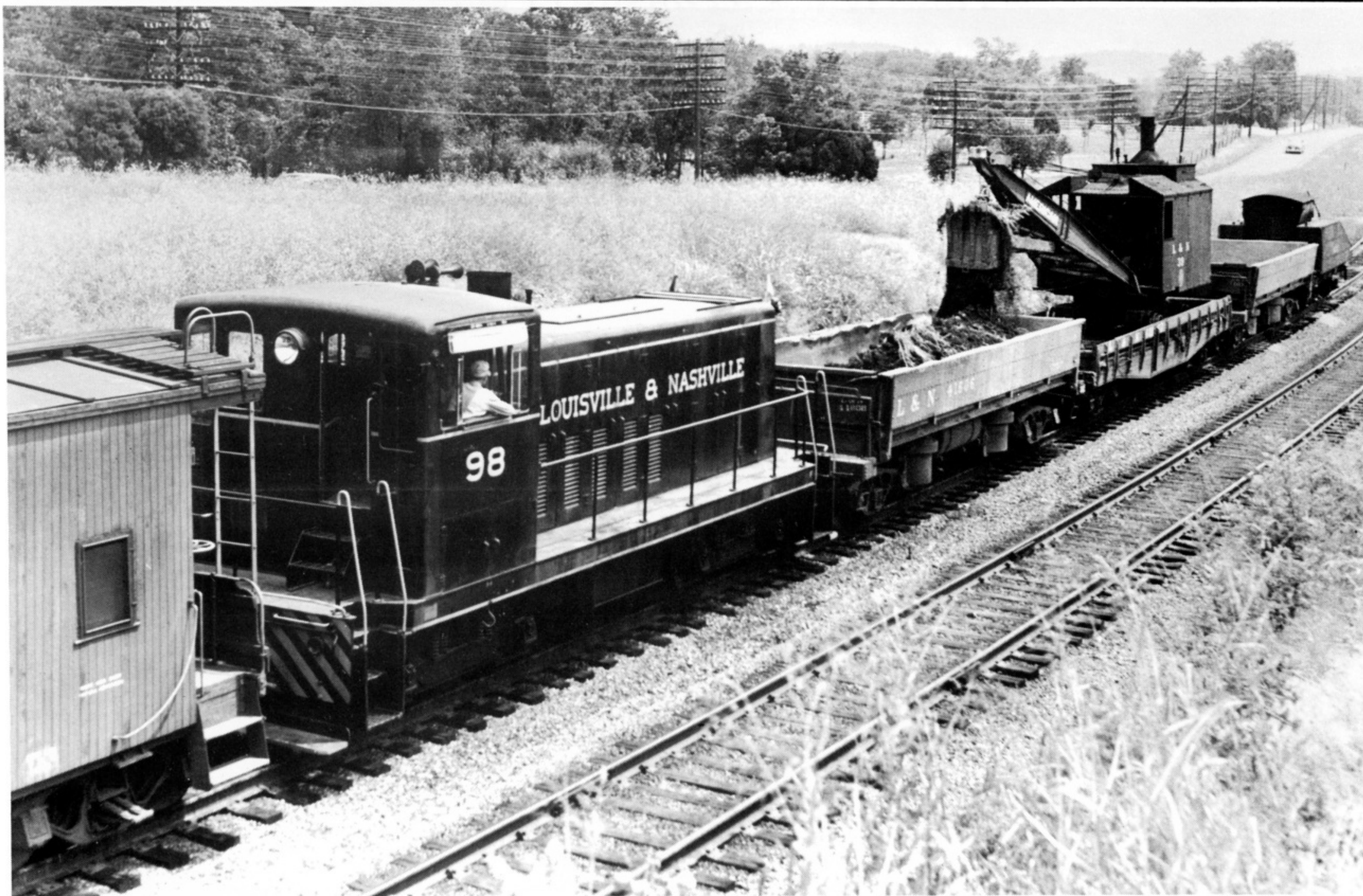
Maintenance of way is the lifeblood of any railroad, and L&N was no exception. On the double track main south of Radnor at Brentwood, Tennessee ancient American steam shovel 39 does some ditching work while GE 70-tonner 98 handles the train. The diminutive locomotive was re-engined with an Alco 251B in 1966 and stayed on the roster until 1980, when it was sold to Tropicana to shuffle reefer loads of orange juice in New Jersey. (J. Parker Lamb)
