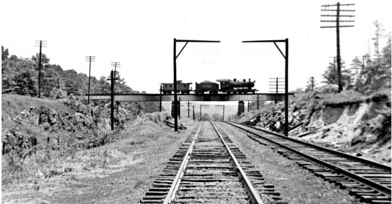
BMRR Red Gap Branch crossing other tracks in Irondale
